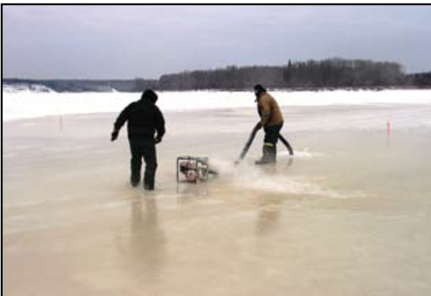
Flooding the ice bridge over the Athabasca River.
